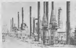
View of Pipesbils 5, 6, 7, 8, 9 and 10.
